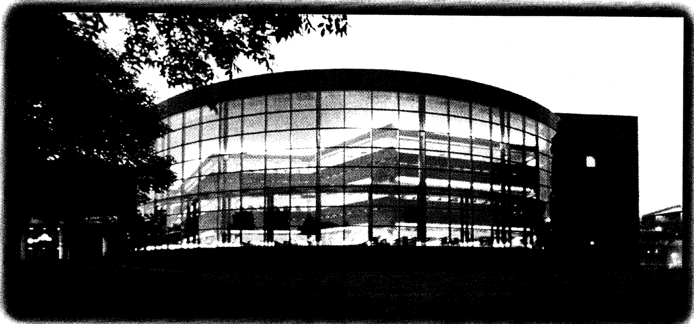
Universal was the electrical contractor for the library at the University of Michigan's Flint campus, a project completed in 1996.
