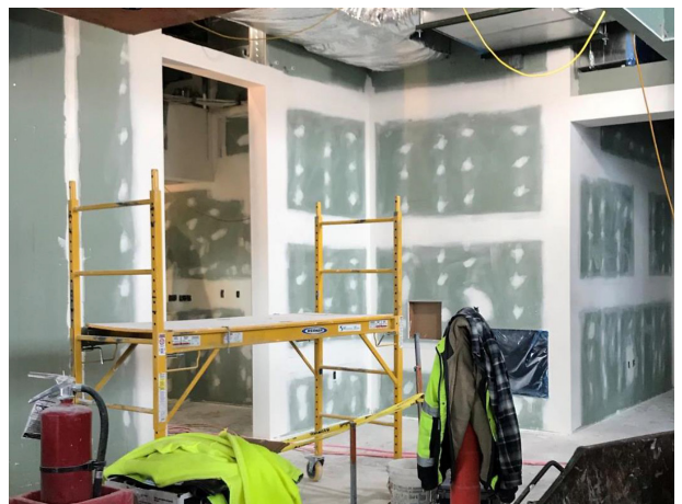
Photo 2. Don't let your job site become an equipment parking lot.
